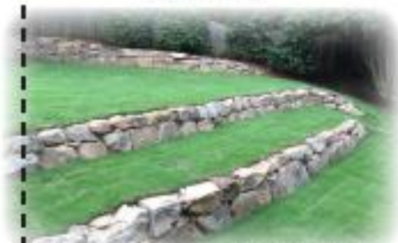
NATIVE FIELDSTONE BOULDER RETAINING WALL
